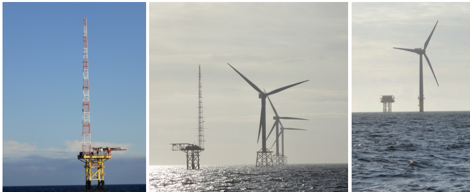
Image C03: Research platform Fino1 (left and middle) close to alpha ventus and relay/transformer station close to alpha ventus wind turbine AV12 (right), taken at 12 th /13 th May 2013.
