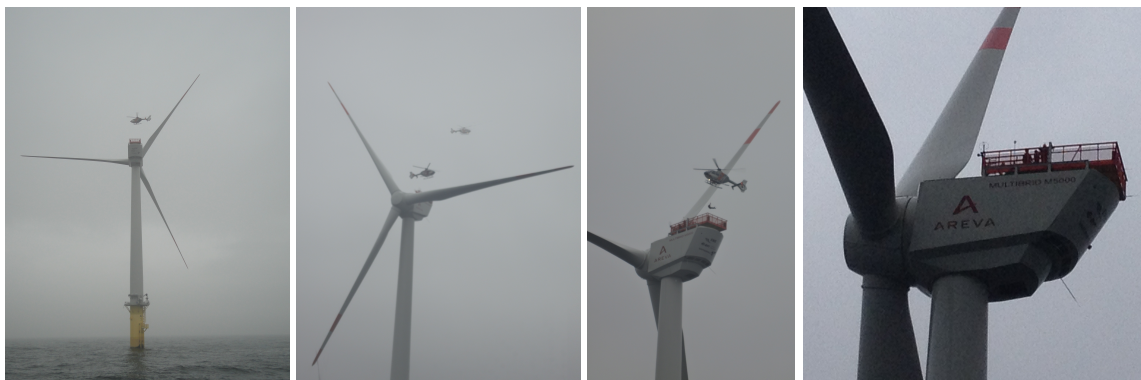
Image C04: Impressions of dimension of offshore wind turbine and nacelle. Helicopters bring people to offshore wind farm and let them down on a rope for maintenance work at wind turbine.
