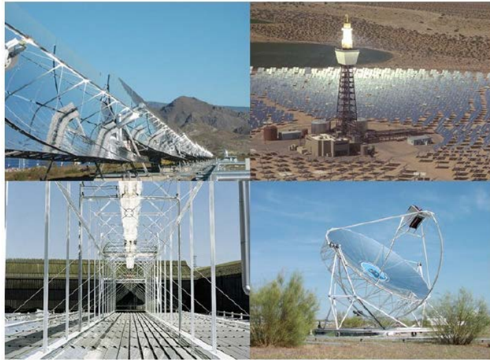
Figure 36: Designs of CSP technology: upper-left is parabolic trough, upper-right is solar tower, lower-left is Fresnel and lower-right is the parabolic dish (Trieb 2005)
