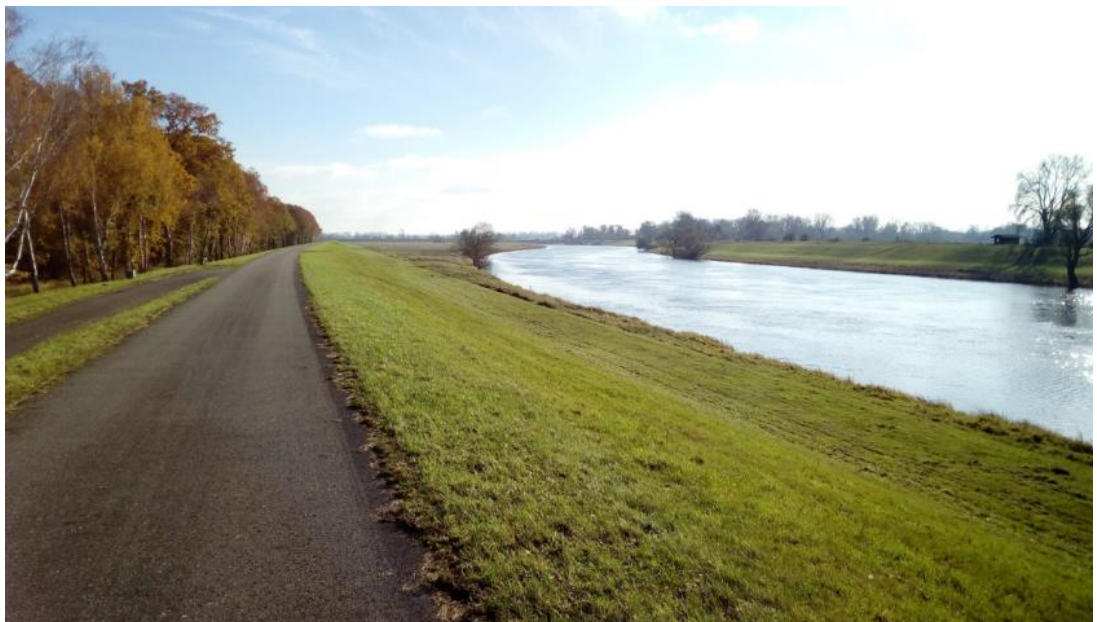
Figure 1.1 Dike presence on the Middle Elbe floodplain constrains the floodplain and alters floodplain hydrology, with the active floodplain besides the river to the right of the dike and the seepage water zone in the former floodplain to the left. Photo taken near Wittenberge in 2018 by Heather A. Shupe.
