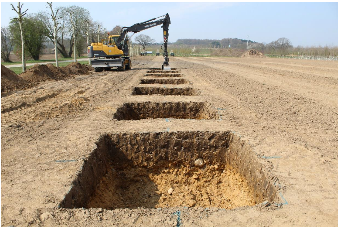
Figure 2.3: Excavation of the first six of the total 135 planting pits in the replication block I. Clearly visible is the brownish Ap horizon and the underlying lighter, but still silty Bv of the horticulturally used Cambisol.
