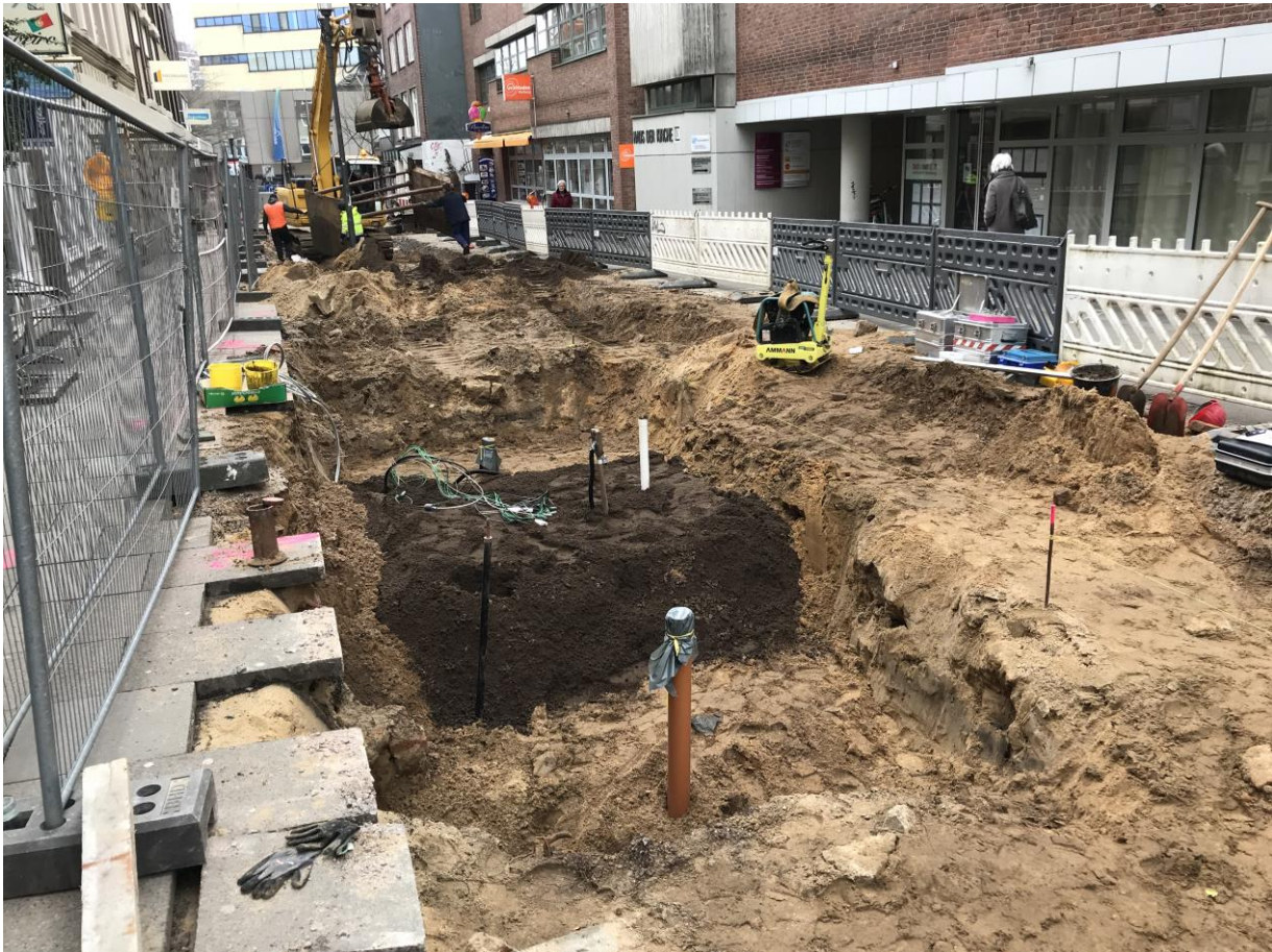
Figure 1.2: View on a future tree site within a pedestrian zone. The excavated planting pit with the backfilled, brownish structural planting soil is located in the center of the zone and is surrounded by the artificial urban soil containing of pure sands.
