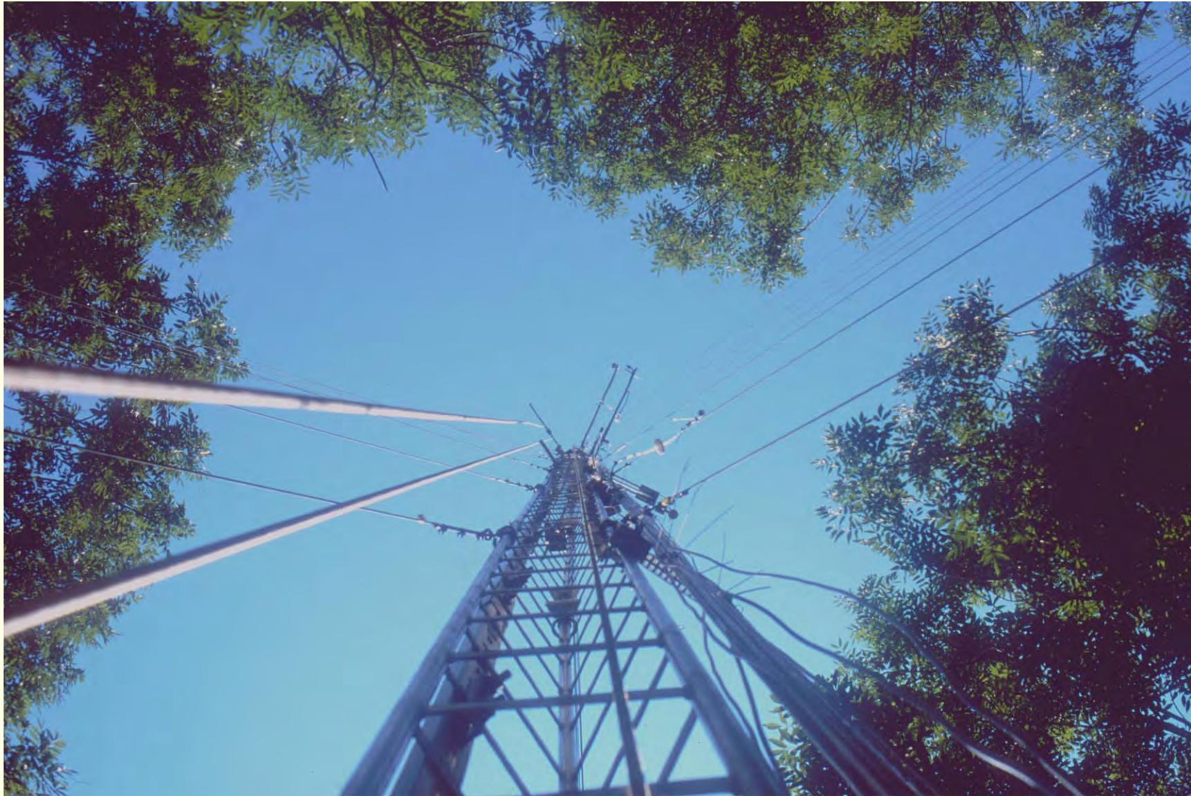
**Figure 3** Hainich Tower from the ground. Notice the booms with the measurement equipments and the inlets for air sampling. Surrounding canopy is from ash trees.
