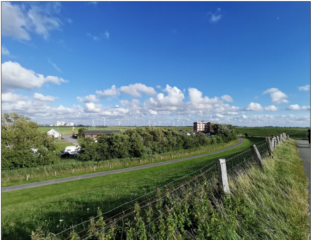
Fig. 12: View towards the Dockkoog with the hotel and campsite in the front and parts of the harbour in the back (own picture, 2020)
