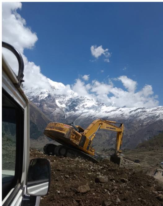
Figure 27 Ongoing road construction work between Nagling and Dugtu
