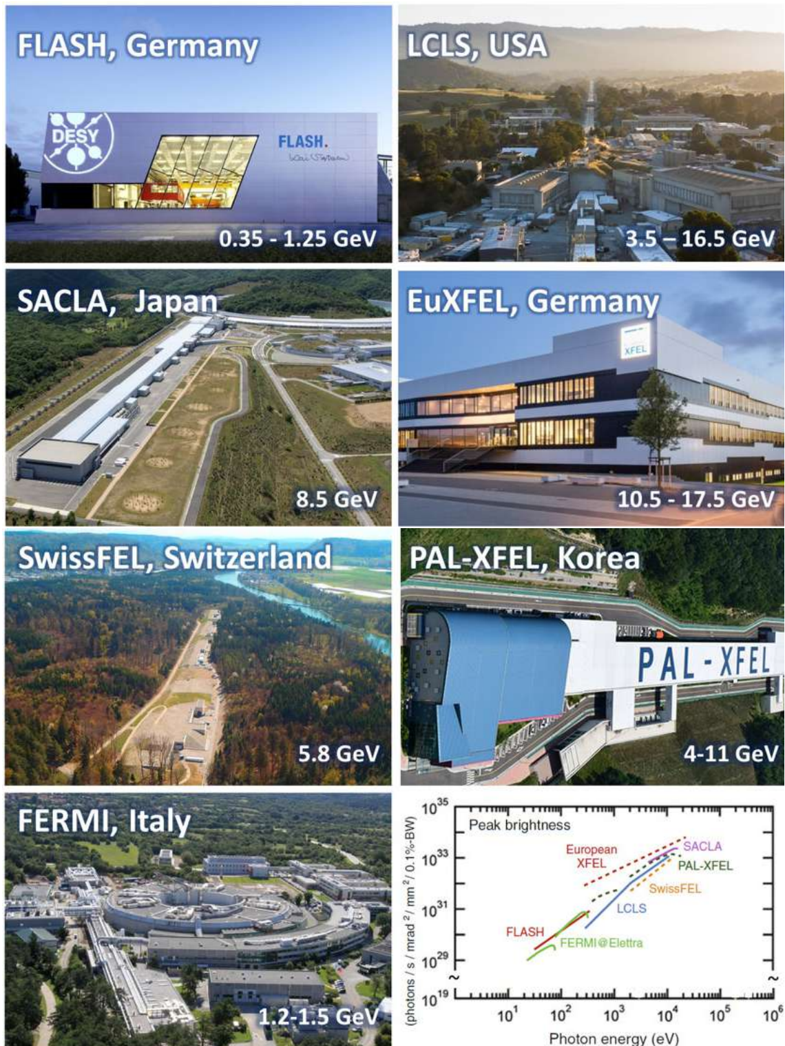
Figure 2.14: Examples of free-electron lasers with a specified electron beam energy parameter that produce soft and hard X-rays. A comparison of the peak brightness of the FELs is displayed in the bottom right plot. Adapted with changes from [15].
