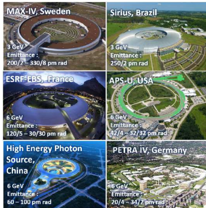
Figure 2.10: Synchrotron sources of the fourth generation that meet the given specifications. Adapted with changes from [21]
