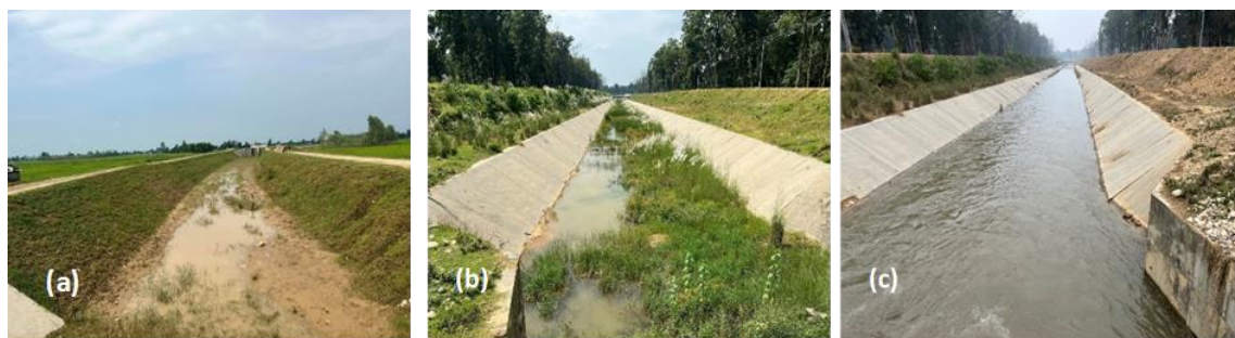
Figure 3-1. (a) Earthen canal with low conveyance efficiency with high seepage and percolation loss , (b) Concrete lined canal but not well maintained with low efficiency, (c) High efficiency well maintained canal lined with concrete.
