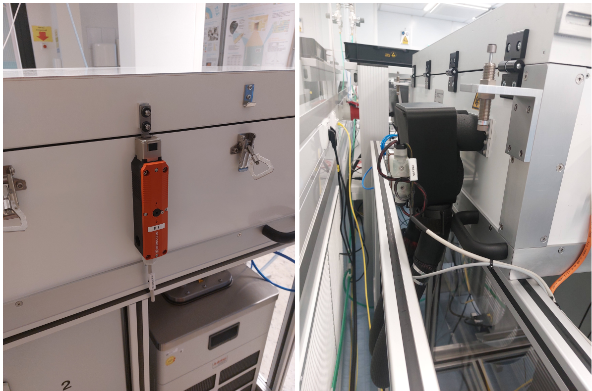
Figure 3.35: Left: coldbox safety interlock. Right: chiller flow bypass.
