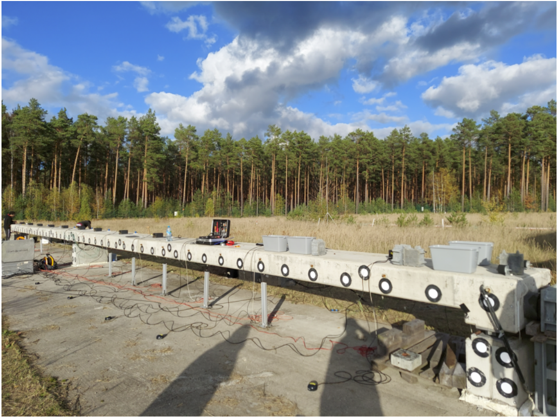
Figure A.2: The placement of the seismic equipment
