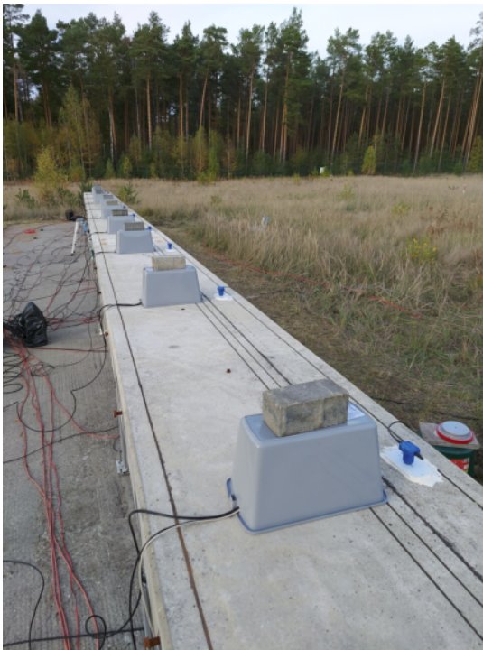
(a) Six-degree-of-freedom sensors covered with grey boxes and one-component geophones attached to the bridge's surface with plaster.
