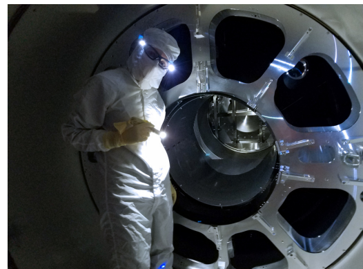
Figure 3.9: Picture of the installation of a baffle in the LIGO beam tube. Image credit: LIGO/Caltech/MIT/Matt Heintze
