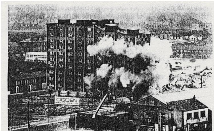
PLATE 1. Failed Utopia. The last wing of a massive complex of flats embodying many officially recommended design features such as 10 storeys poised on concrete stilts, internal corridors, flat facades and flat roofs. When built, a brochure was circulated to local authorities showing it as a Utopian ideal to be imitated. Yet it proved unsalvageable and hundreds of imitators were also condemned to a short life. (Eldon and Oak Gardens, Birkenhead)
