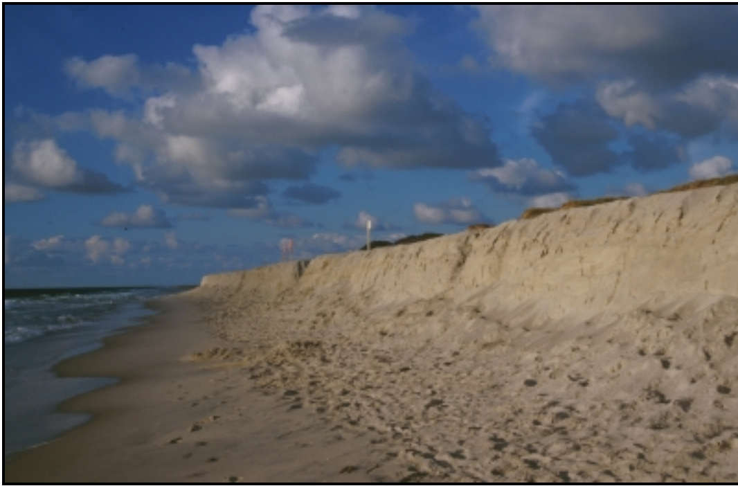
Fig. 9 Nourished sediment forms a new cliff on the beach of approximately 2.5 to 3 m depending on the volume of nourished material (island of Sylt, Germany).
