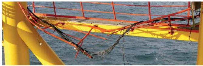
Fig. 4. Steel-bridge at the FiNO 1 research platform damaged by ocean wave crest 18 m above normal sea level (source: German Weather Service, DWD).
