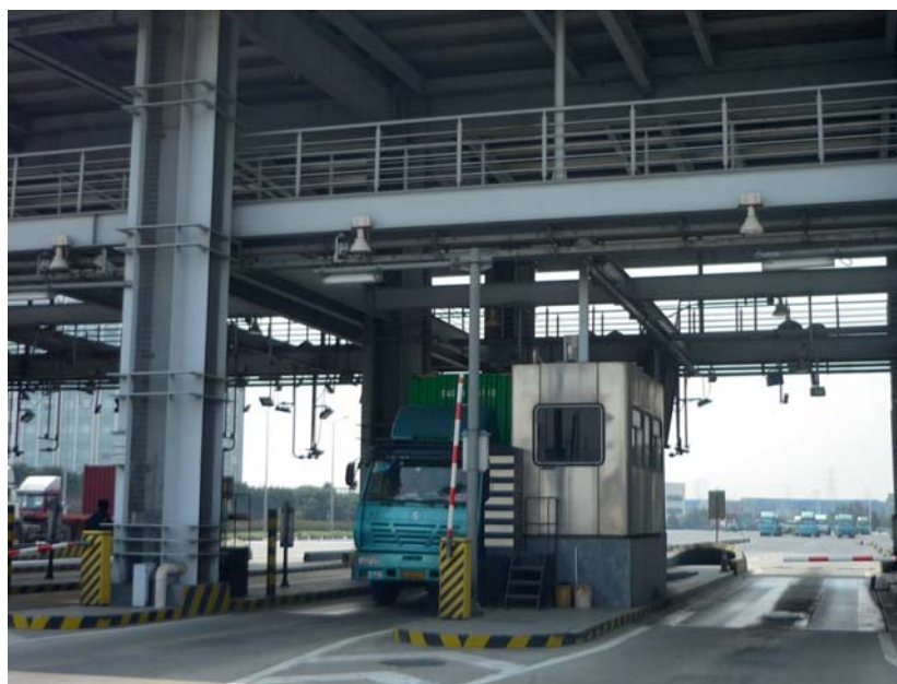
Figure 1 RFID application at entrance gate of container terminal (color figure available online).
