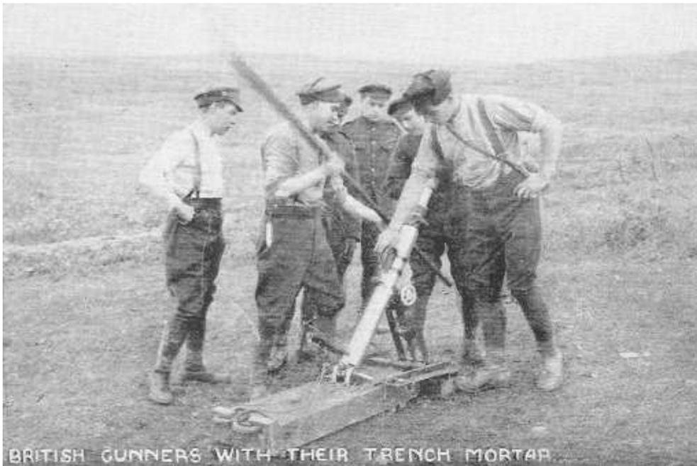
Abb. A3.7.: Vickers 2 inch Trench Howitzer Mark I,
