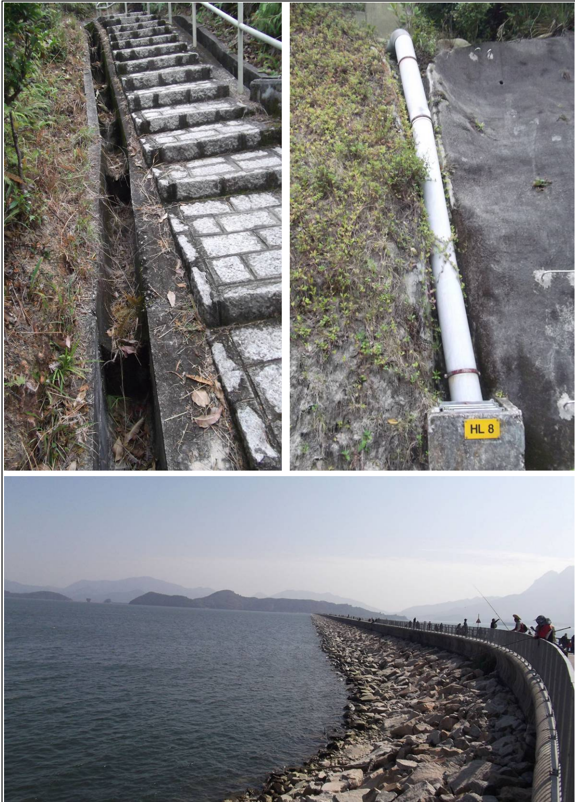
Figure 3-8 Photographs of the rainwater collection channels in the Lung Fu Shan Country Park (top two), and the Plover Cove Reservoir (bottom), Hong Kong.
