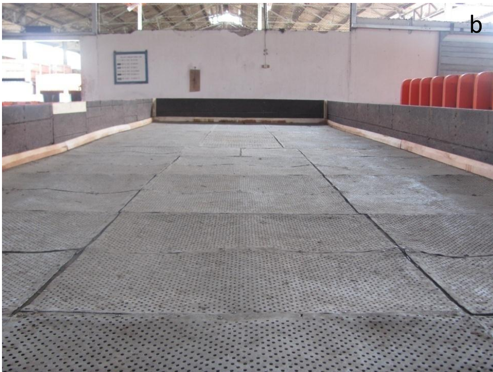
Figure 1.9 Artificial drying facility with a capacity of 4500 kg, a) view from outside, b) view from inside in Nusantara Plantation XII (PTPN XII), Jember, East Java, Indonesia
