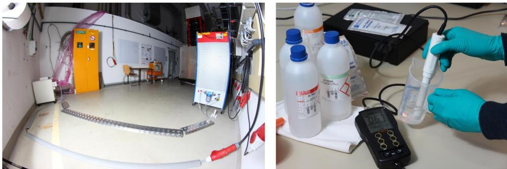
**Figure 2.8: Water cooling system status after January 2015** - On the left, picture of the water circuit including the compressor and the chiller taken with a fish eye objective. On the right, picture of the EC/T/TDS/pH meter. (Source: Y. Berger)
