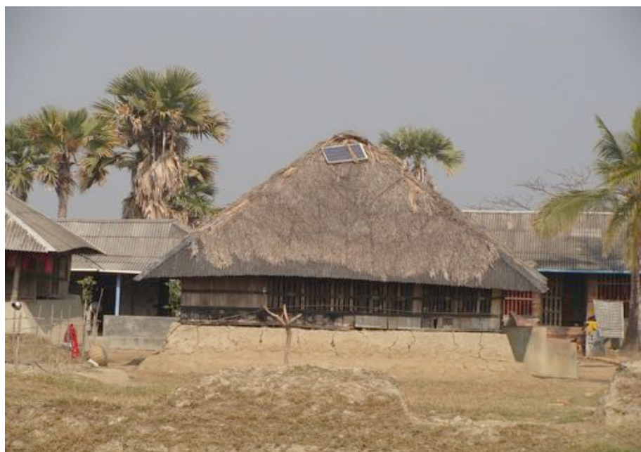
Figure 3.4: A common house structure made of local materials in Gabura village. A solar panel is visible on top of the thatched-roof (researcher's own photo).
