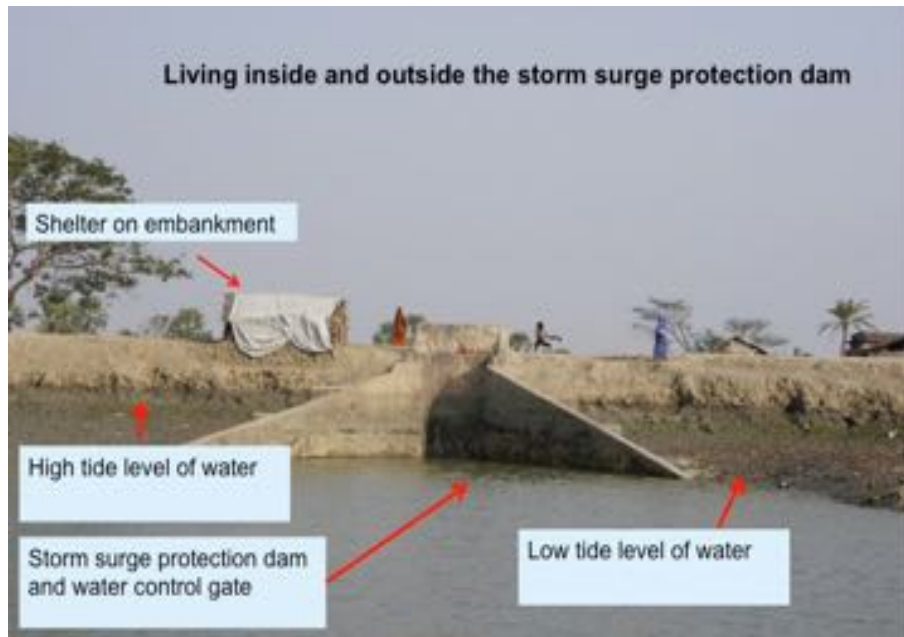
Figure 3.3: A mud-built dike to protect the villages from intrusion of saline water during the times of high tides and storm surges (researcher's own photo).
