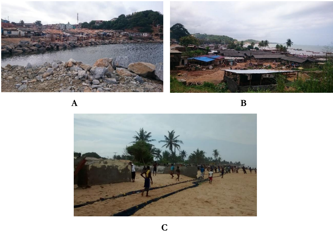
Figure 4.7: Selected photos of the coast of Ghana showing sea defence structure at New Takoradi (A) ; Coastal settlers relocate close to the sea at Ngyiresia after a flooding event (B) ; Community members pulling in a fishing net at Blekusu (C) .
