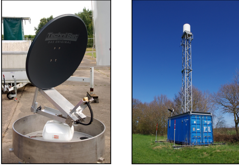
Figure 2.2: LAWR device without radome (left) showing the parabolic antenna and as installed at QNS site (right). It is mounted on a 11 m mast fixed on a 3 m high container.
