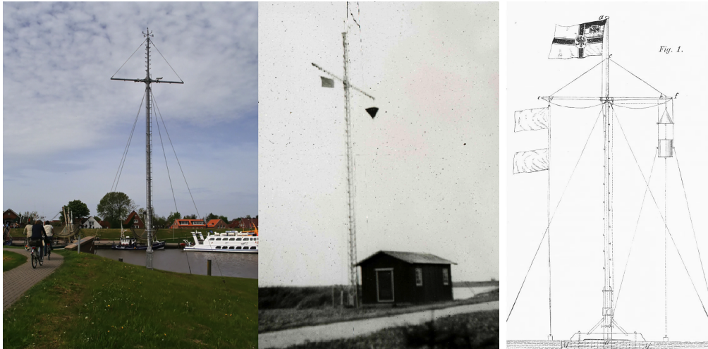
Figure 2.1.: On the left side, a picture of the signal mast in Greetsiel and in the center the signal mast in Karkeln (Poland) before 1945 with optical signals. On the right side, a detailed drawing of a signal mast with optical signals. Source: DWD.
