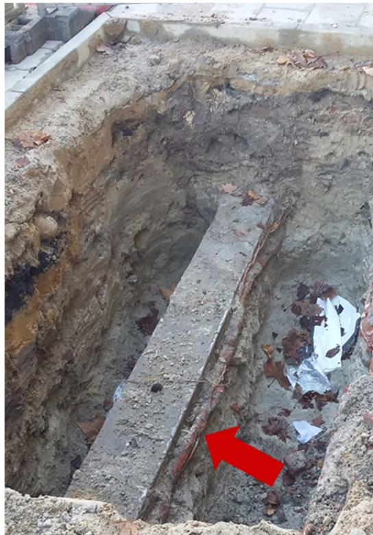
Fig. 6.2 Tree root of a not identified tree species growing along a cable duct below a sidewalk in the city center of Hamburg. The distance to closest mature trees was ~20 m. (Photo by Volker Kleinschmidt)
