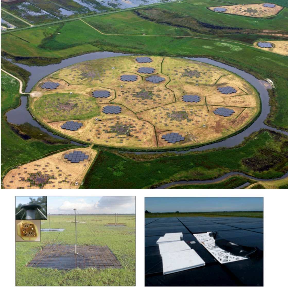
Figure 1.13: Top panel: aerial photograph of the Superterp: the circular island encompasses 6 core stations (CS). Additional CS are visible in the upper right and lower left of the image. Each of them includes 96 LBA and 2 sub-stations of 24 HBA tiles each. Bottom left panel: a single LBA dipole including the ground plane. The inset images show the electronics in the cap and the wire attachment points. Bottom right panel: a single HBA tile, showing underneath the protective covering where the dipoles are located. Credit: images adapted from van Haarlem et al. [2013a] .
