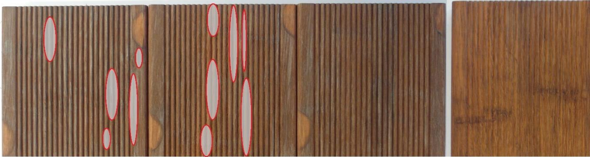
Figure 87: Naturally weathered samples of commercial bamboo scrimber (left) with the reference (right) and severe longitudinal cracks on the surface (red ellipses)
