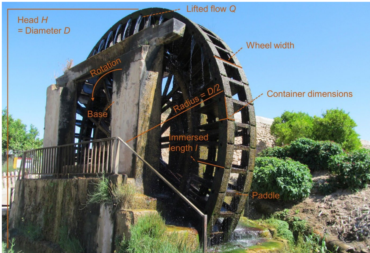
Figure 4.4 Geometric and hydraulic characteristics of norias (here: Noria de la Hoya, Abarán)
