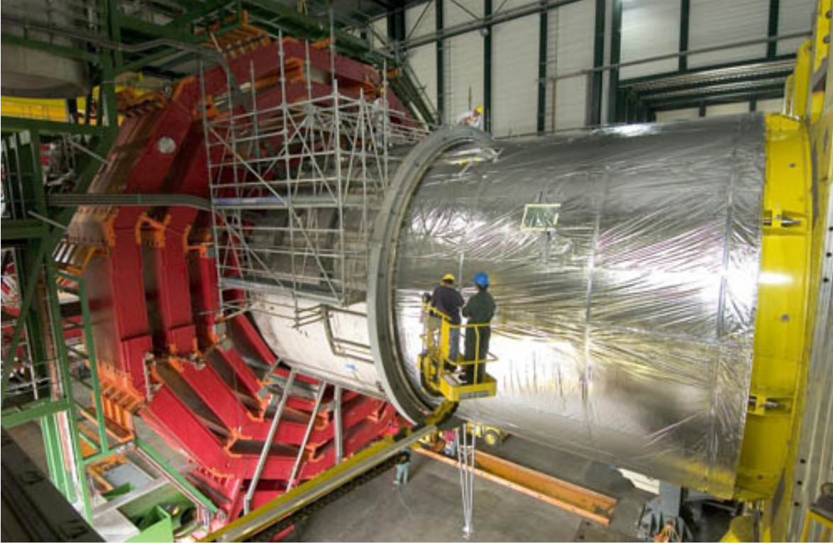
Figure 3.8: The CMS magnet during construction. The cylindrical magnet coil and the return yoke (12-sided red structures) are shown (this figure is taken from [90]).
