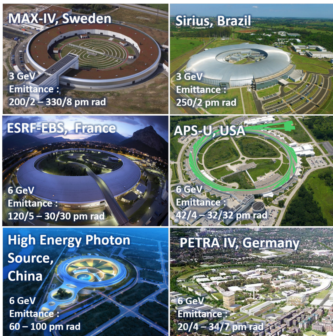
Figure 2.5: Examples of the 4 th generation synchrotron sources with the specified parameters.
